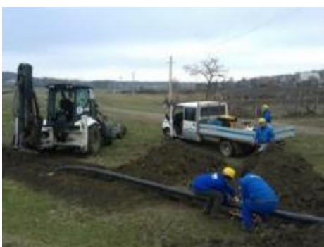
Works in progress
